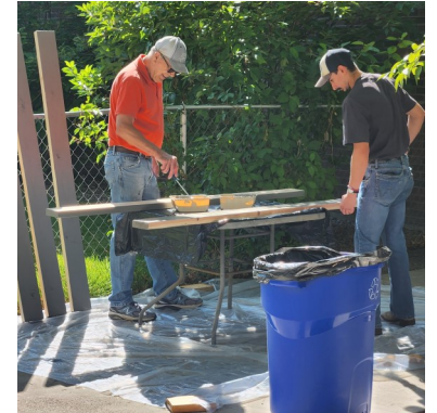
Warren Johnson and Mathias Pepos stain boards for Bethel Patio.
